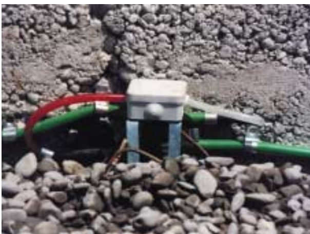
• Sealing of joints between floor/wall by PREDIMAX ®
