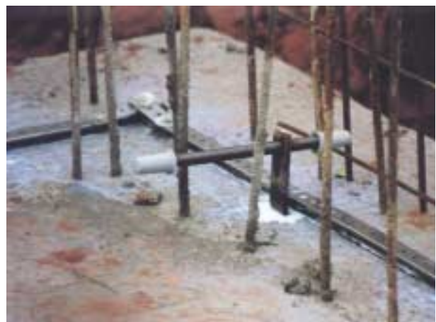
• Sealing of joint between floor/wall by QUELLMAX ®
